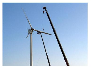
The cost for replacing a gearbox in a 660 kW turbine, on a 65 meter tower, is on the order of \$120,000, for a site with local hydraulic crane service. The bulk of this cost, perhaps 80%, is for procuring and overseas shipping the new gearbox, and the remainder is for crane, site labor and local shipping. Overhauling the gearbox at a local rebuild shop can reduce the total replacement cost to around \$40,000 - \$50,000; these facilities are
